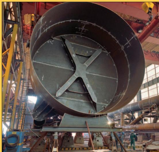
Four 9m diameter suction cans provide the seabed foundation for the barge.
