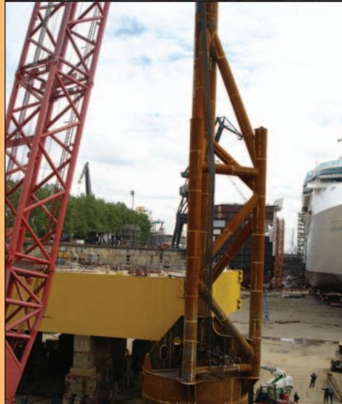
1500t barge substructure being built around the hull.
