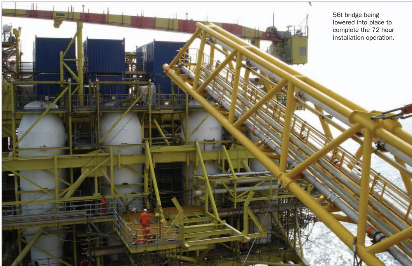
56t bridge being lowered into place to complete the 72 hour installation operation.
